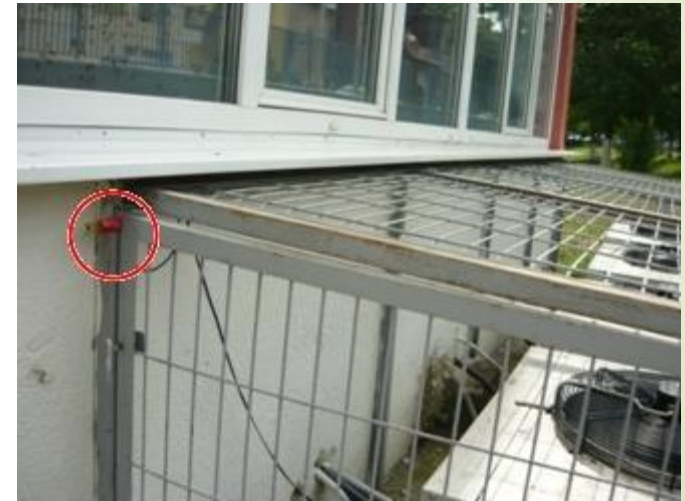
The temperature sensor for the environment outside of the cooling system
