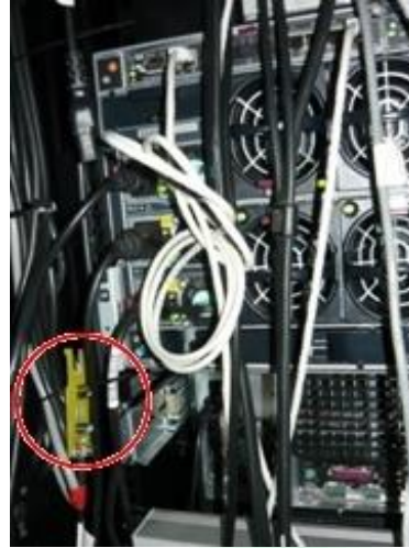
Temperature sensor in hot areas inside the servers rack
