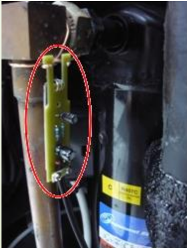
Temperature sensor on cooling agent pipe of air conditioning system
