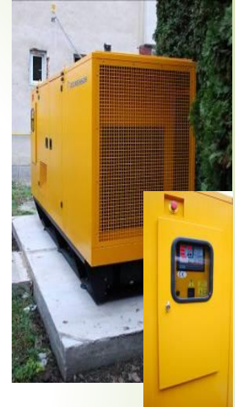
Power generator 275kW
